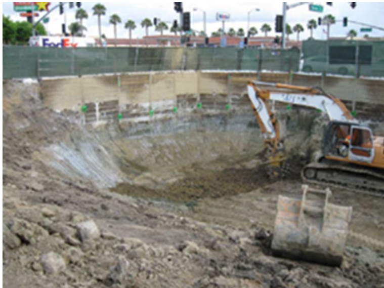
Figure 3. Soil excavation site.
